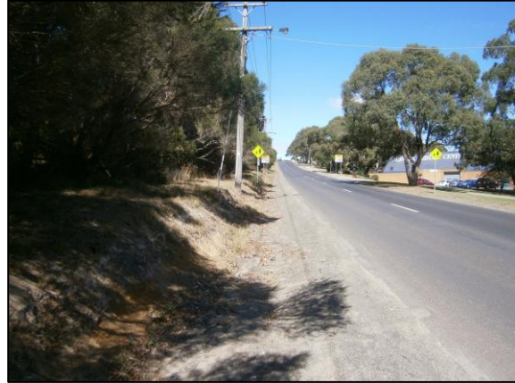
Figure 4: Manuka Road - View South
