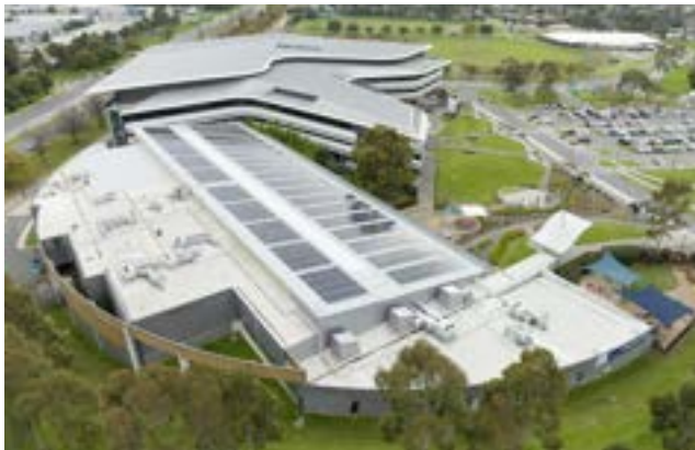
340kW rooftop solar system on Casey ARC, Narre Warren.
