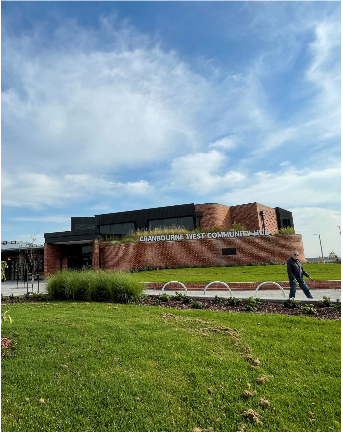
Image: Cranbourne West Community Hub, Cranbourne West
