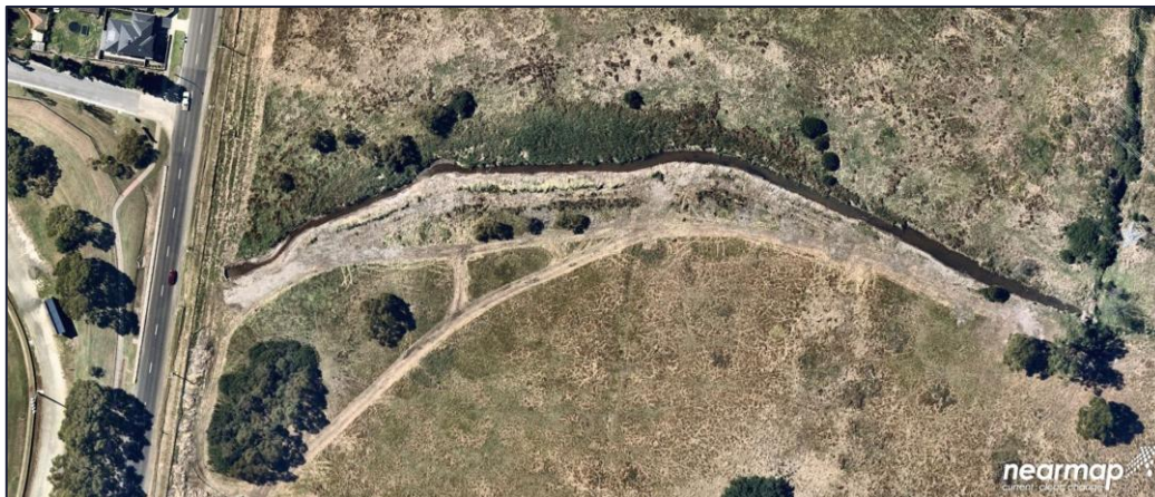
Figure 4-5 Nearmap – Cleaned swale (February 2022)
