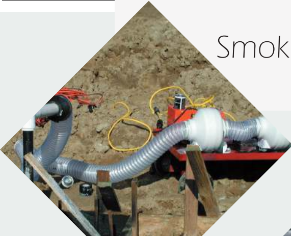
Equipment set-up for smoke test
