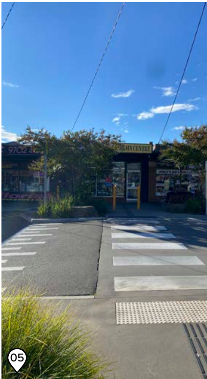
Raised pedestrian crossing prioritises pedestrian movement and improves safety at key crossing points.
