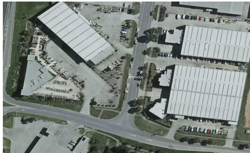
Lynbrook Industrial estate, despite space requirement for truck movements, shows significant opportunities to improve tree canopy cover along existing nature strips and walking paths.
