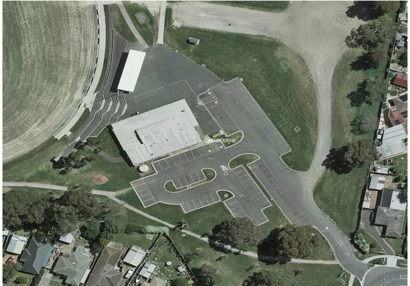
J and P Cam Reserve Carpark has 0% tree canopy cover providing great opportunity for improvement.
